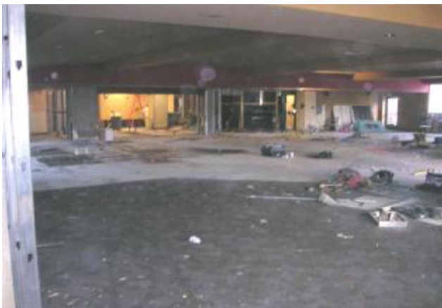
Scottsdale DWR during demolition of restaurant space
